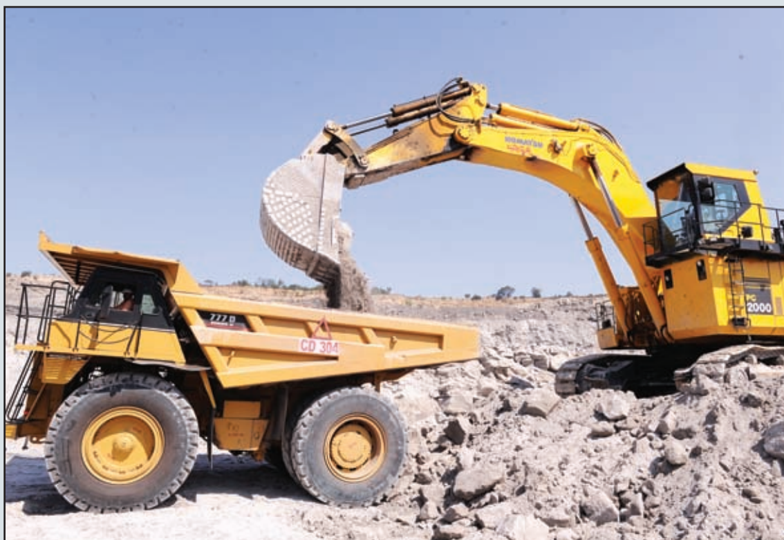
Over burden removal by Shovel & Dumper combination
