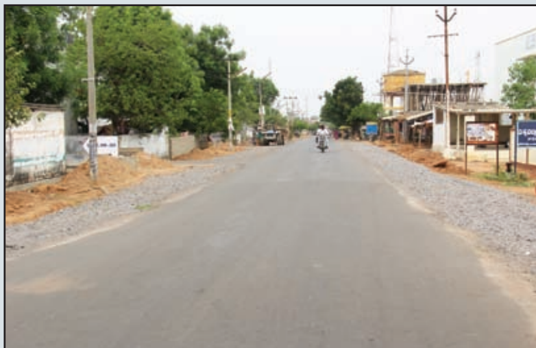
D T Roads laid as part of CSR activity in surrounding Towns and Villages - A view of a road in Bhupalpalli town
