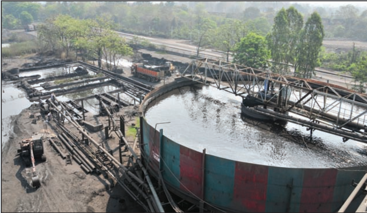
Coal washery at Manuguru area for supply of clean and washed coal to customers
